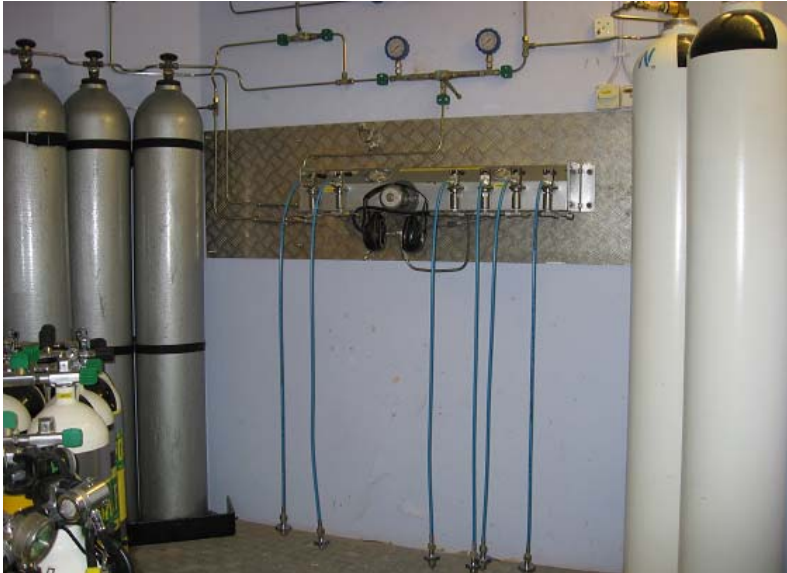
Figure 3. Filling station for diving air.
